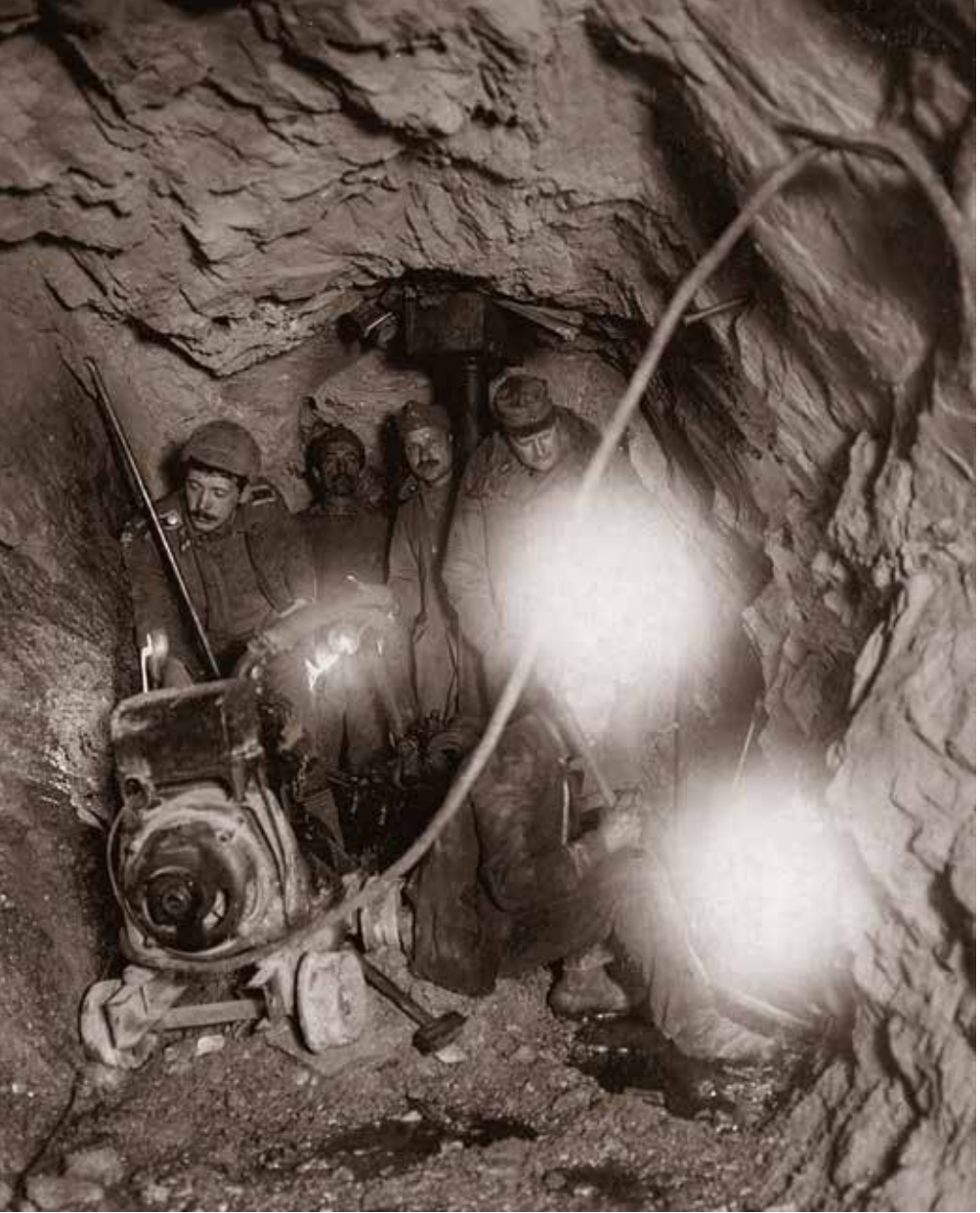
Forward extension of a gallery using a drill press, Imperial and Royal Gravel-Ore Mining, Großfragant, around 1916.
