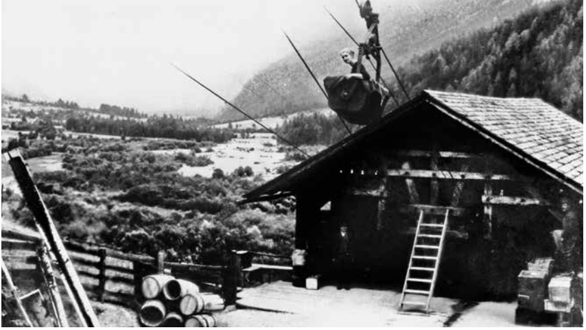
Cableway Grafenberg–Außerfragant, around 1915. Photo: Austrian Alpine Association, Klagenfurt
