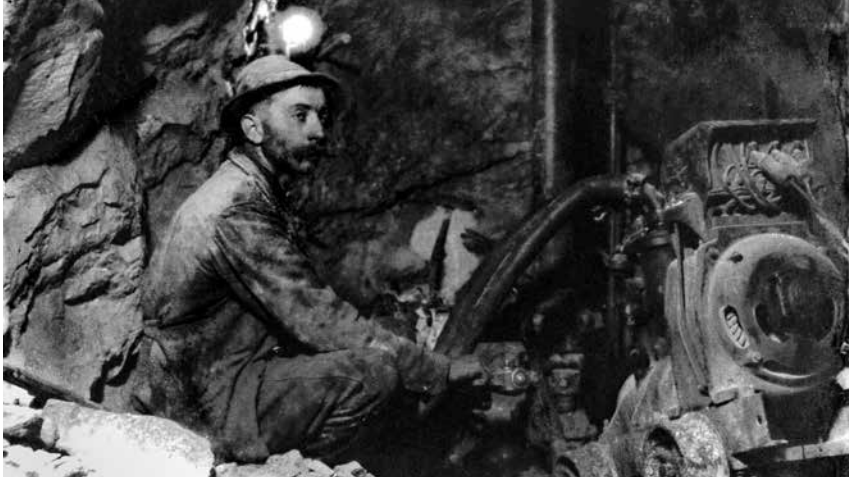
Gallery workmen, Großfragant, around 1915.
